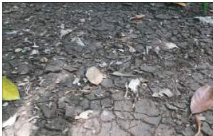
Fig:4.2. Deposited silt (Soil Survey and Conservation, 2018)
